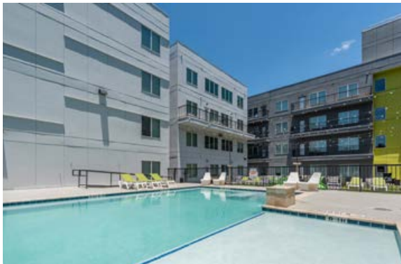
ELLA LOFTS 75 UNITS | 252 BEDS | YOC 2016 TEXAS STATE UNIVERSITY | SAN MARCOS, TX
